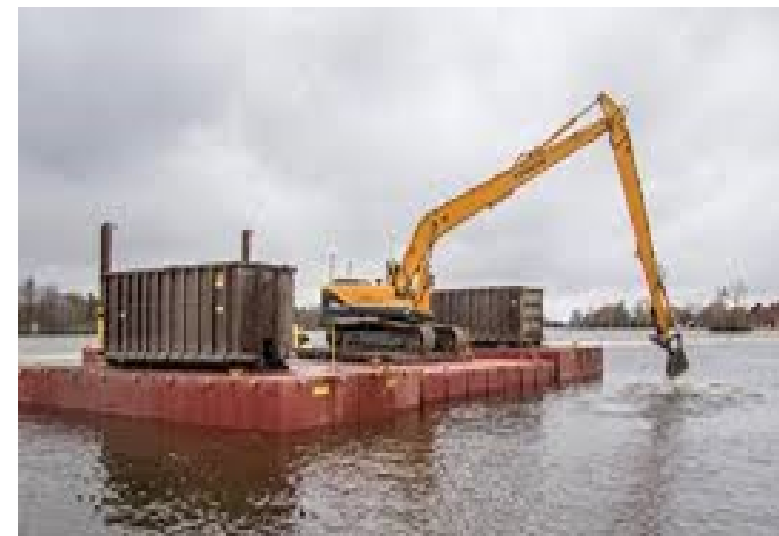
Mechanical Dredging Water Based
