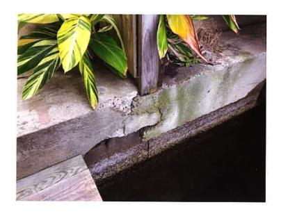
**Symptoms:** The principal symptoms are rust, spalling, exposed rebar, and fractures.
