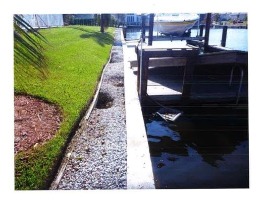
**Symptoms:** Sinkholes upland of the wall, visible back-fill mounds in the water near bulkhead joints (most visible at low tide).
