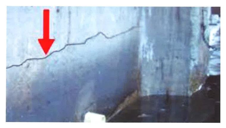
Note horizontal crack at mid-point of concrete panel – the weakest point of the seawall, particularly at low tide. Crack is likely caused by either excess hydrostatic pressure or possibly a tieback failure. Drain (bottom of picture) was likely installed in response.
