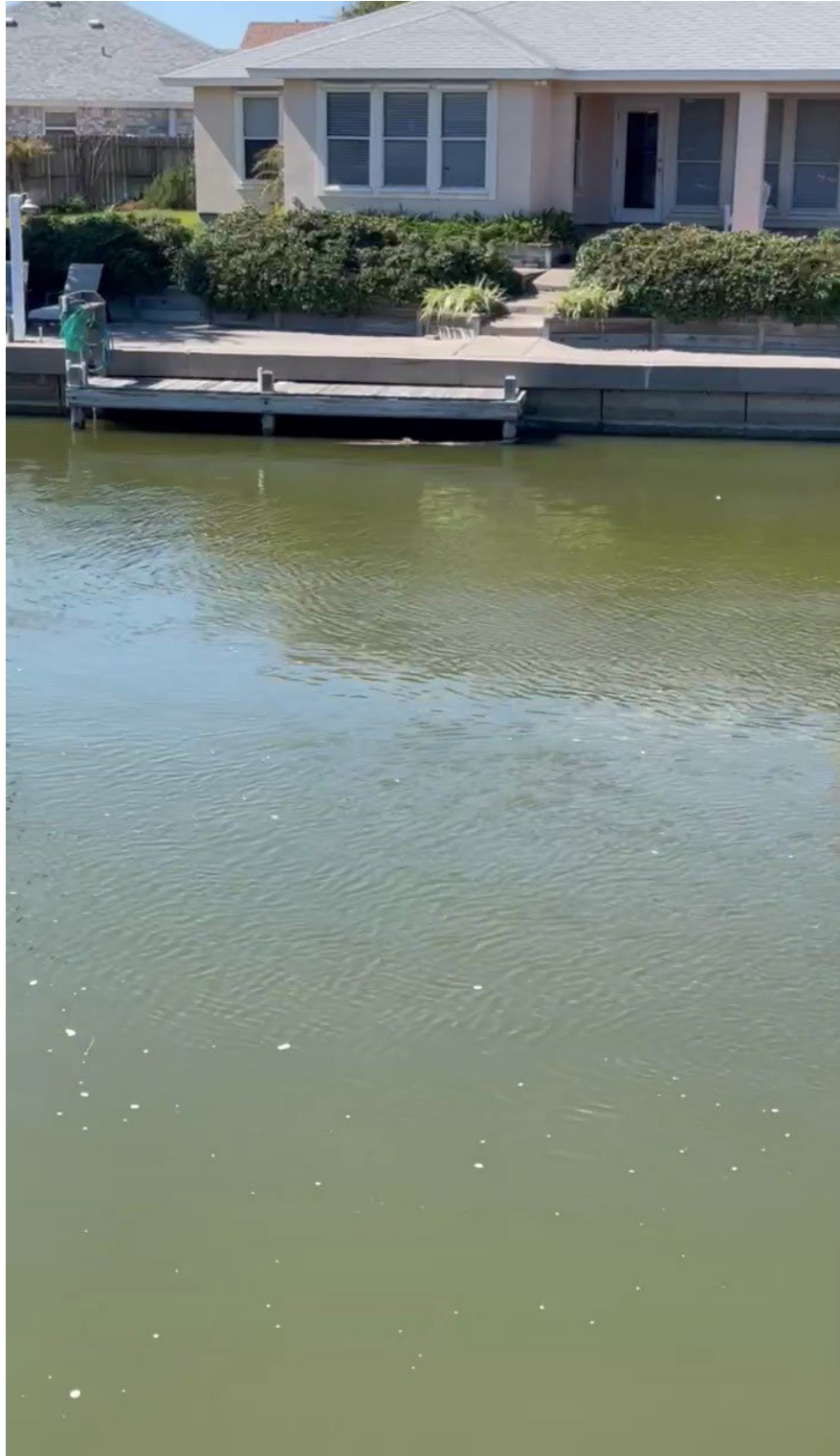
Figure 1 Canals Partially Open 18 Feb 24
