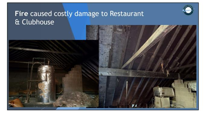
You can see here part of the HVAC system, and you can see part of the firewall – note how it does not extend all the way up. \*\*This means we must treat both buildings as one as far as occupancy permitting is concerned
