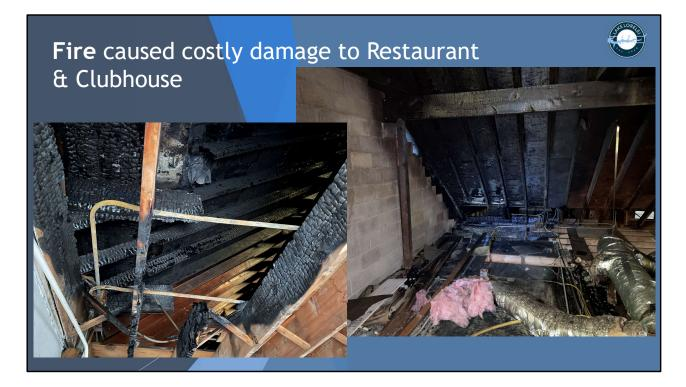
This is the roof above the Restaurant You can clearly see here the damage to the roof beams and rafters, and associated electrical, plumbing, and HVAC that runs through it
